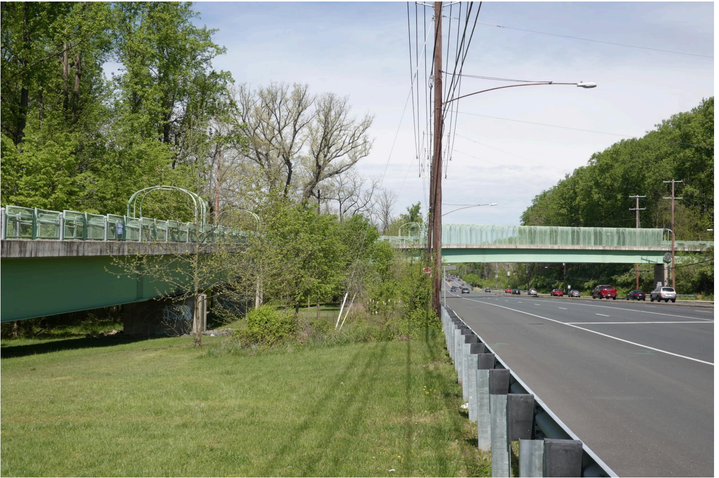
Rock Creek Trail Bridge over Veirs Mill Rd.
