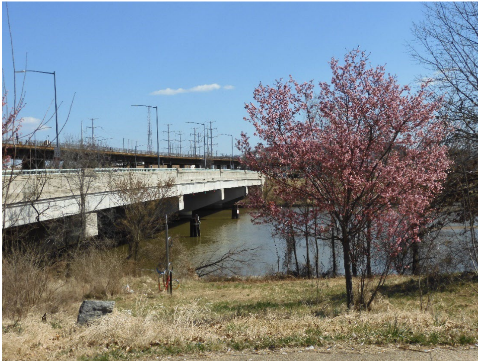
Figure 5 View of Benning Road Bridge
