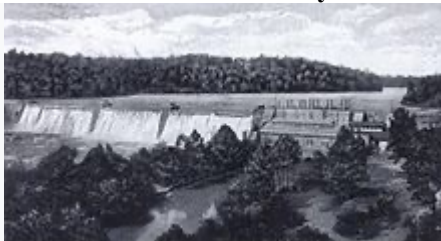
Portman Shoals Power Plant around 1920.
