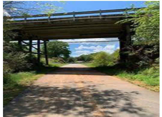
Figure 1: overhead bridge at Ireland Rd.
