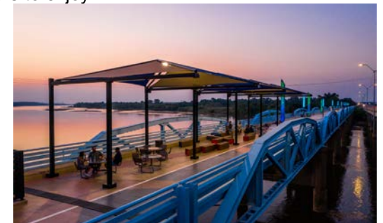
Bixby Harmony Bridge
