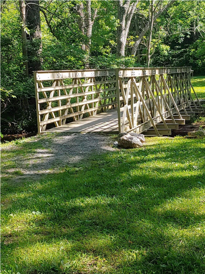
Bridge over Little Bennett Creek (5K and 10K).
