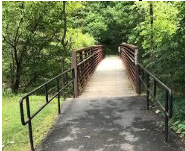
Bridge at Start Point
